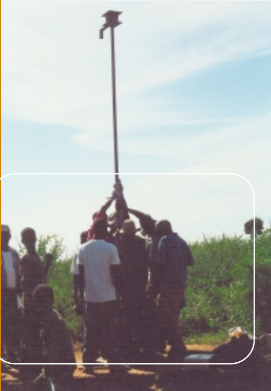
Lifewater-trained Haitian crew installs the new pump.
