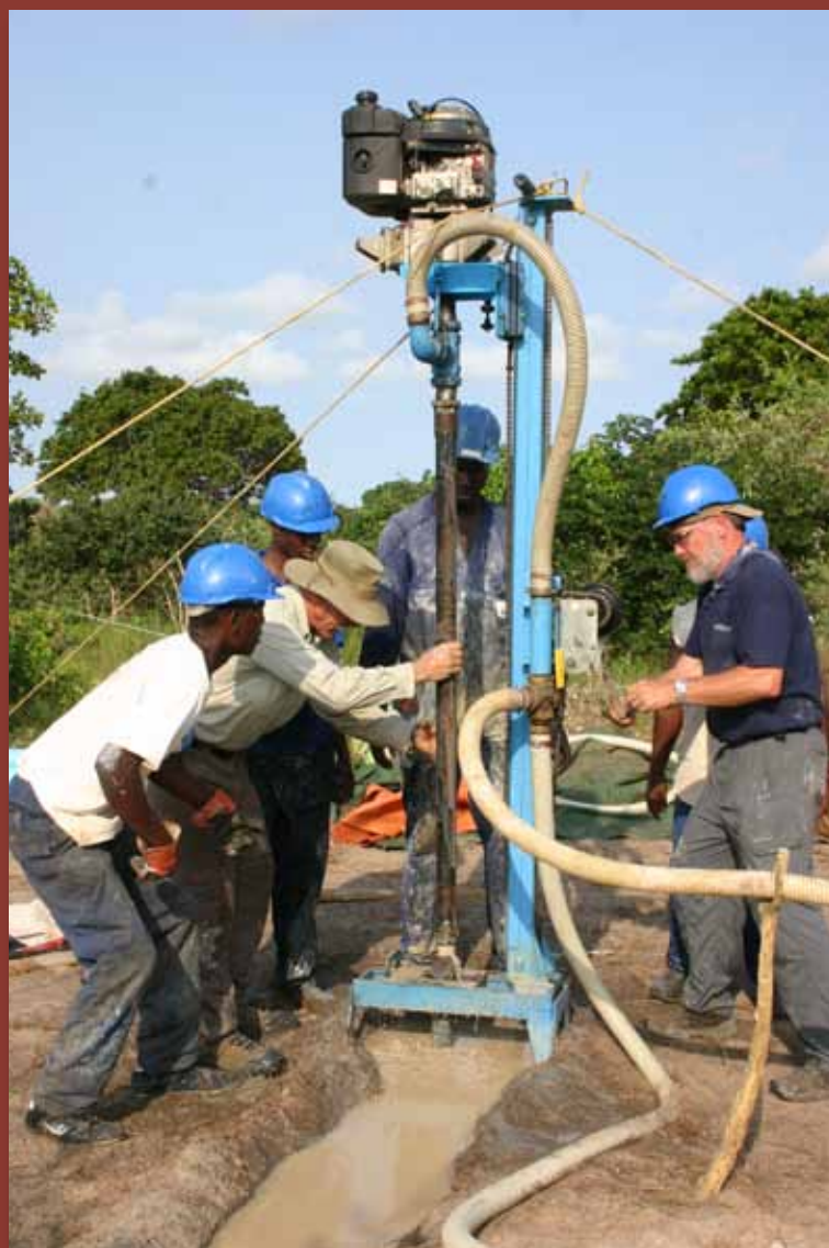
Lifewater staff and field trainers teach shallow well drilling to in-country partners. Photo by Shawn Roberts, field trainer
